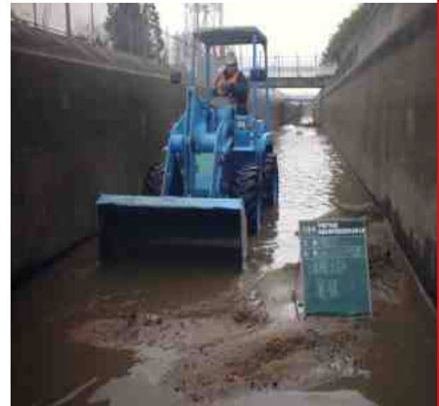
Removal of silt and sediment
