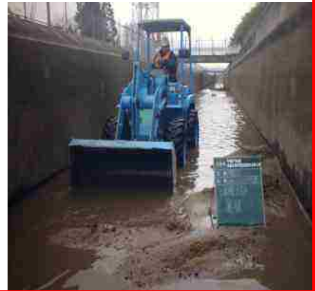
Removal of silt and sediment
