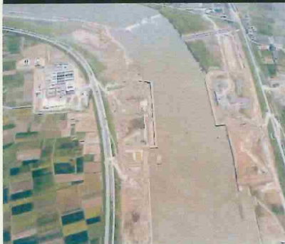
First stage construction work (December 1980 to September 1981)
