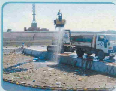
2 Unloading refuse with back-hoe
