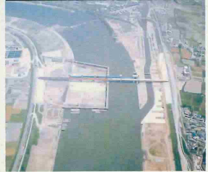
Third stage construction work (October 1982 to May 1983)
