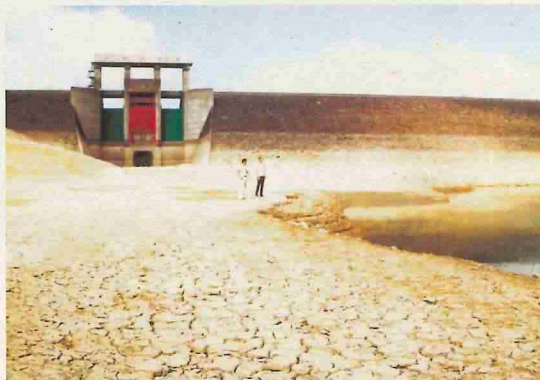
The water shortages in 1994 (Terauchi Dam)
