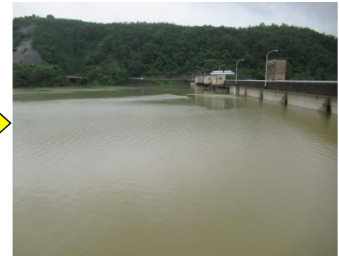
State of the reservoir with water approaching the maximum level during flooding (Approx. 17:00 on July 6; EL.150.81 m (water continuing to rise))
