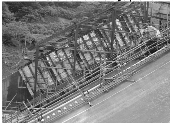
Photo 3. Construction of a Training Wall with Large Sliding Forms
