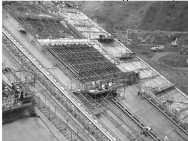
Photo 2. Construction of a Training Slip Forms
