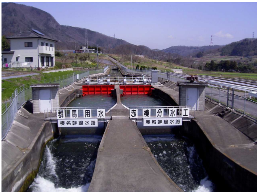
Sekisin Division The water dividse Left: Akagi main canal Right: Haruna main canal
