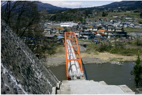
Agatsumagawa siphon (Akagi main canal facility)
