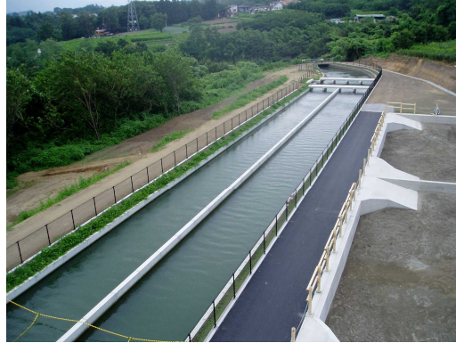
Hassaki open canal (Haruna main canal facility)
