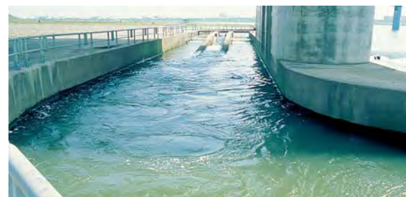
Attracting-flow-type fishway at high tide
