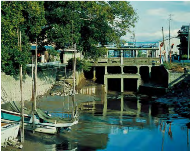
A basin gate used in the old method for obtaining fresh water
