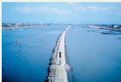
Water transmission embankment near river mouth
