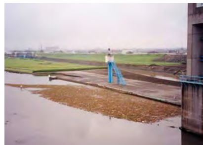
The refuse clogging the locks interferes with the passage of ships and the movement of fish
