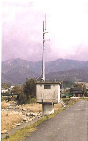
Water level observation station There is one station at both Agi River and Iwamura River and another two stations in the dam downstream area to observe water level automatically.
