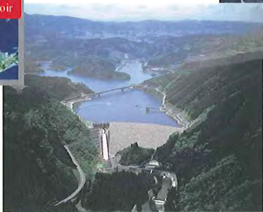
Agigawa Dam (Completed in 1990)
