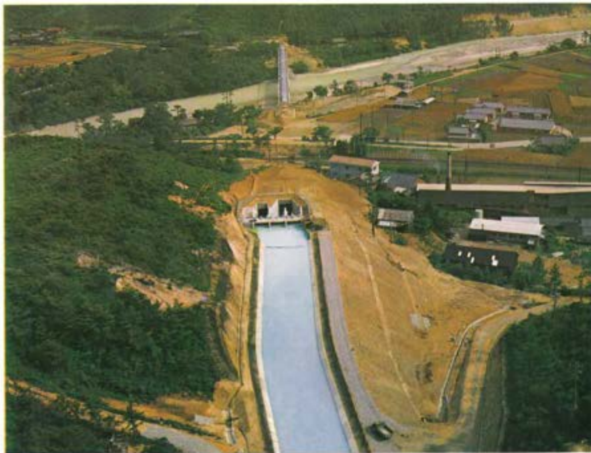
The entrance of Kozoji Siphon and Steel Pipe Bridge seen from upstream side.
