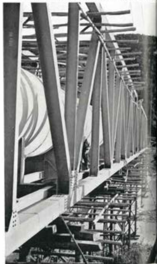
Steel Pipe Bridge under construction.
