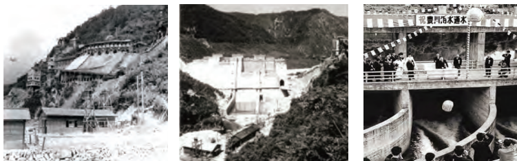
Water transmission commencement ceremony held at Ohno Head Works on 30th May 1968.
