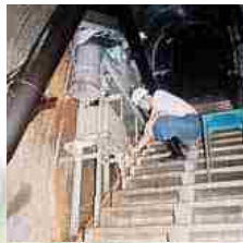
Measuring leakage (inside of inspection tunnel)
