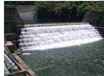
Yugakegawa sediment dam
