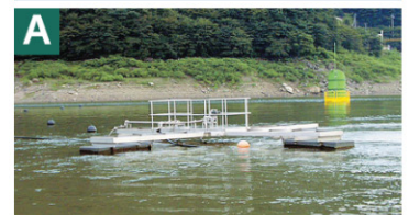
A Epilimnion derating and recirculating equipment Four sets are installed at location A.
