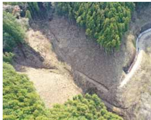
③付替林道西ノ入下流1工区工事 (R1.11.19~R2.9.3)
